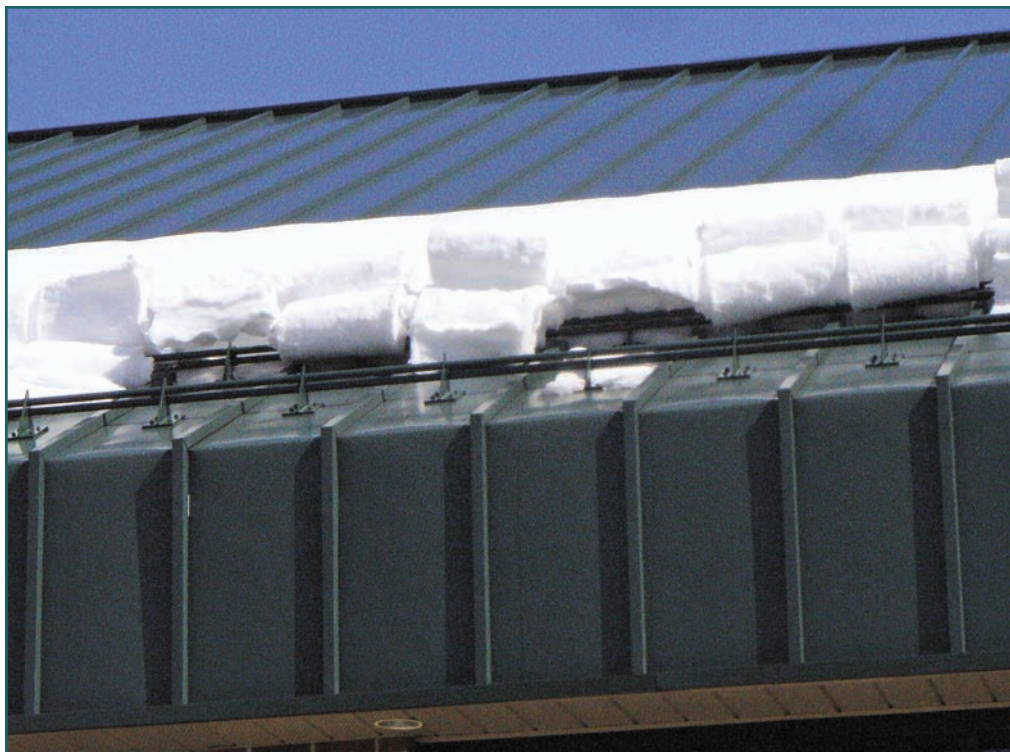
Photo 2 – Bar retention system.
