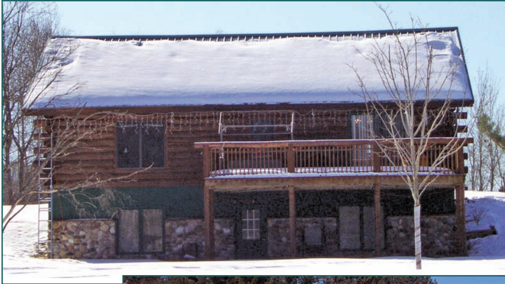
Photo 14 – Green snow retention coating on 10/12 pitch. A snow slide in a prior winter tore the railing off the deck.
